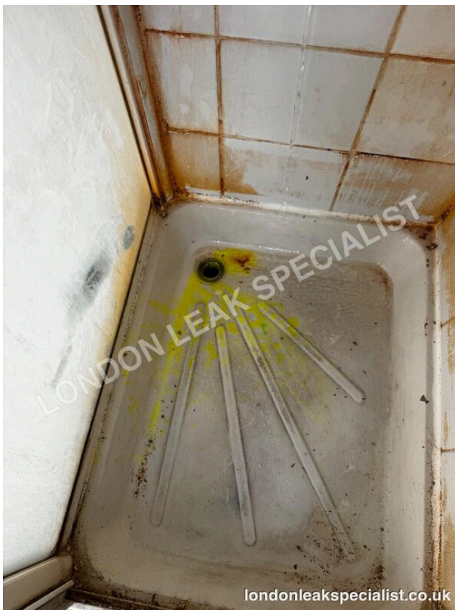
Photo 3. Yellow tracer dye run into a shower tray waste during the waste pipe test.
