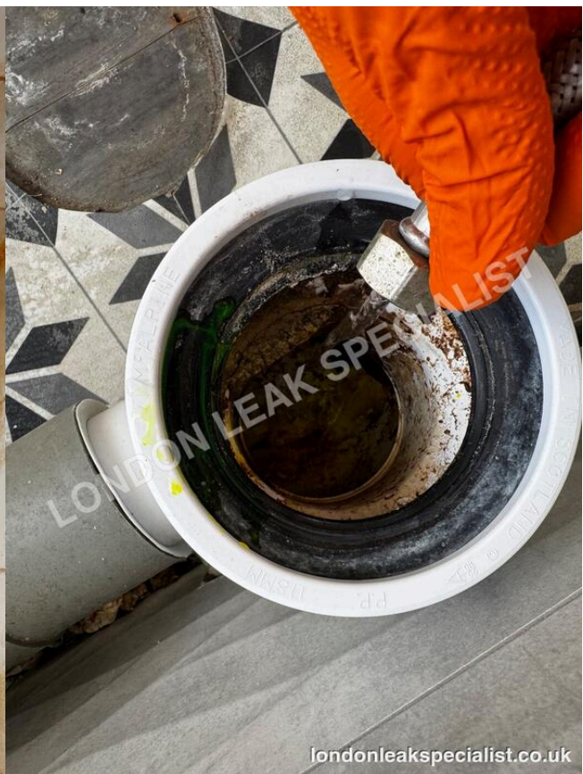
Photo 4. Tracer dye being introduced at an open waste outlet.
