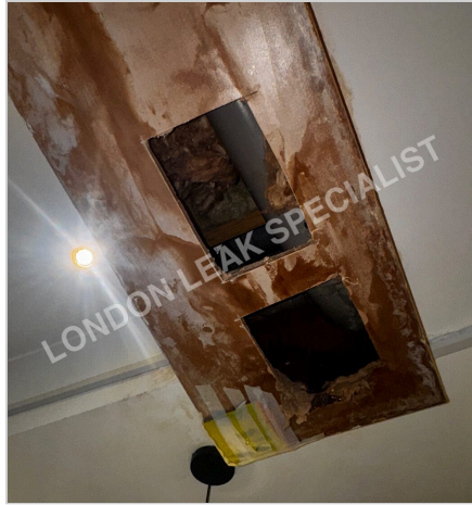
Inspection openings in the boxed-in ceiling section below
