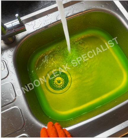
Tracer dye test: the upstairs kitchen sink filled with warm dyed water
