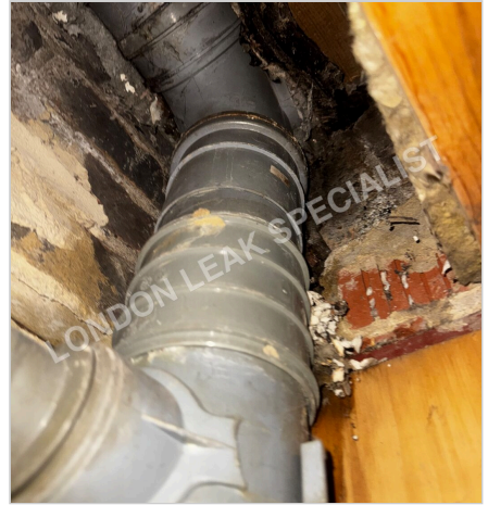
The main soil and waste stack exposed in the ceiling void
