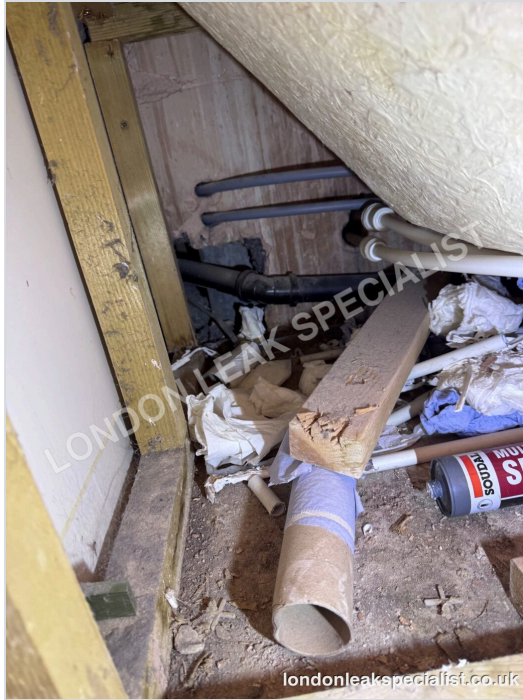
Photo 5. Targeted access beside the bath showing the supply and waste pipework.
