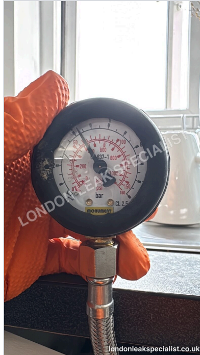
Photo 1. Pressure gauge connected to the isolated supply during the hot and cold pressure tests.
