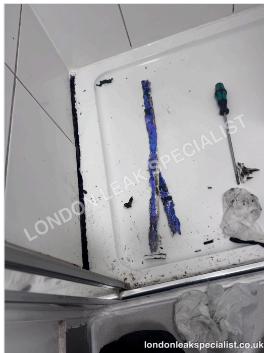
Photo 4. Blue tracer dye from the earlier visit, found in the tray void.
