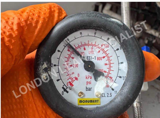
Photo 3: Pressure gauge during the cold-water test
